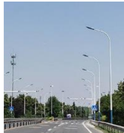
Protected Street Lights
