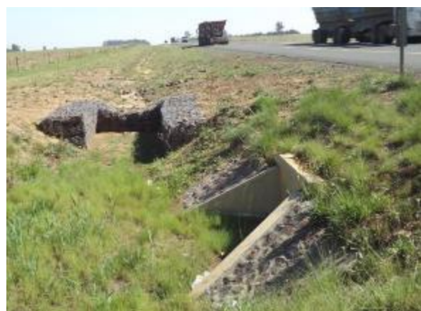
Inlet structures within clear zone
