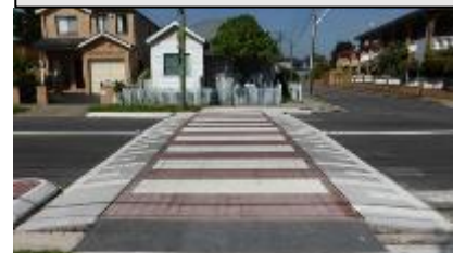
Raised Pedestrian Crossing
