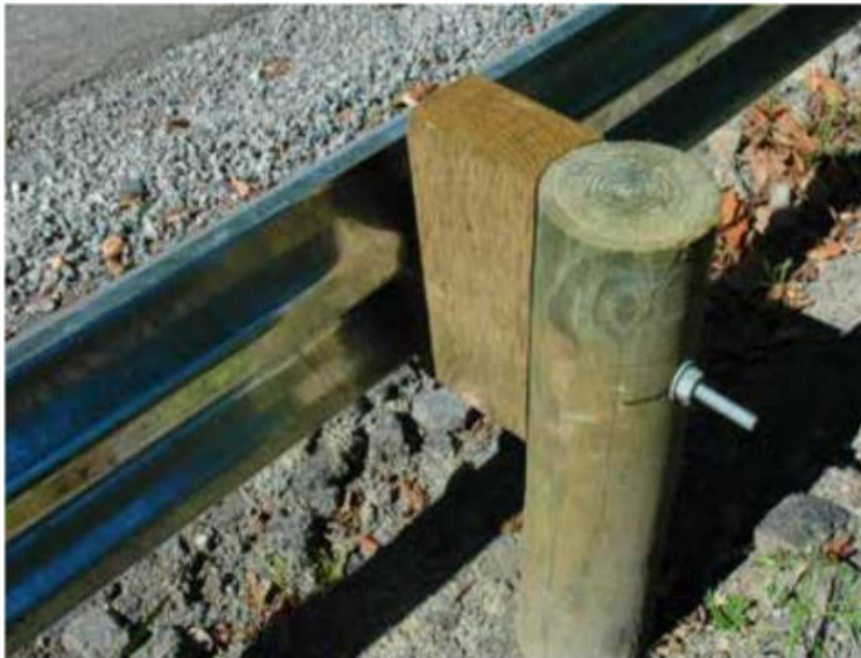
Figure 15: Illustration of Post and Beam Connection
