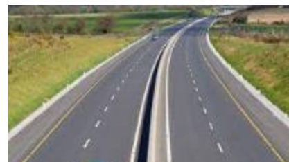
Well maintained horizontal curve
