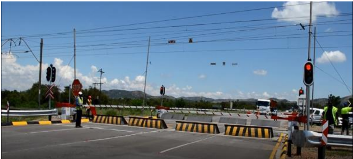
Figure 36: Boschhoek Railway Level Crossing with Barriers
