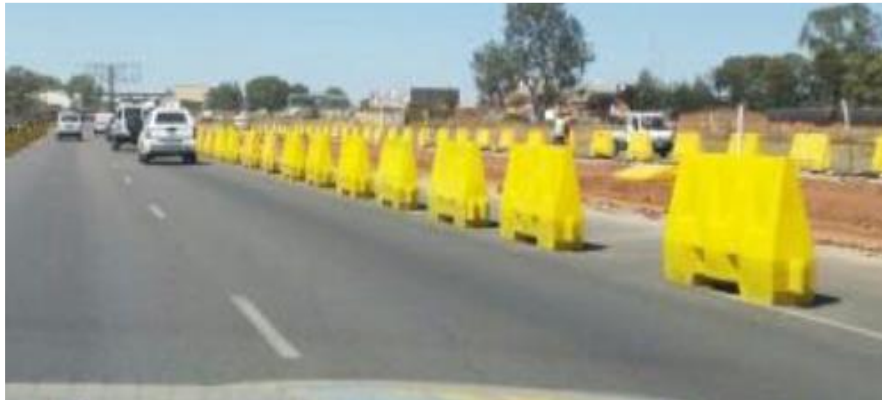
Figure 34: Yellow Plastic Units Used as Delineators
