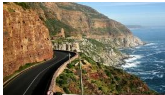
Stone Masonry barrier on Chapmans Peak Drive
