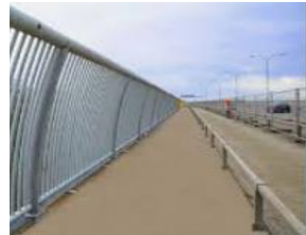
Protected pedestrian walkway
